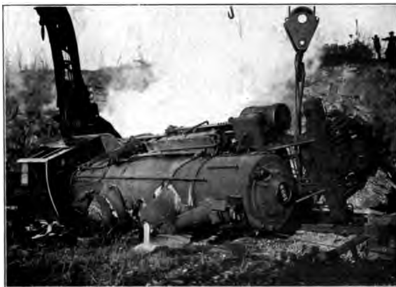
"TWO OF THESE GREAT CRANES CAN GRAB A WOUNDED MOGUL LOCOMOTIVE AND PUT HER OUT OF THE WAY"
